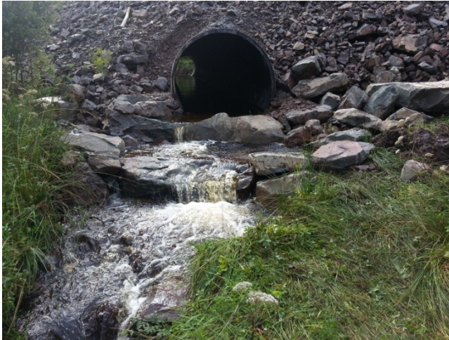
Fig vi fish pass in forestry culvert
